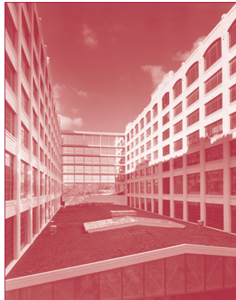
Example of an Extensive Green Roof System—Montgomery Business Park/Maryland Department of the Environment, Baltimore, Maryland.
