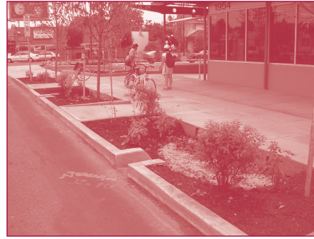
Example of on-street bioretention areas—Portland, Oregon.
